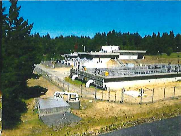
Photo3: LPCD Outlet Works & Treatment Plant
